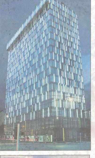
LEFT: The Power Tower in Linz is the first high-rise office building built with passive-house characteristics. The building draws energy for heating and cooling from the ground and a solar power station on the south-west façade generates electricity.
